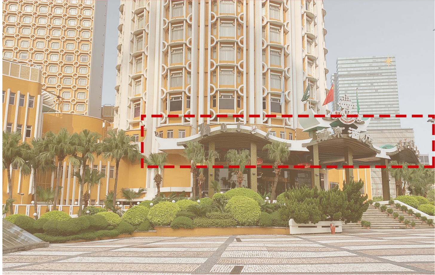
Figure 33. A bat shape canopy in the main entrance. (Author, 2020)
