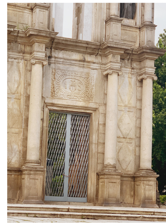
Figure 6. First floor entrance. (Author, 2020)
